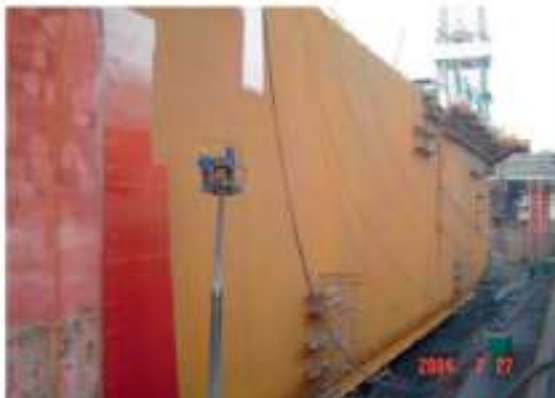
Figure 1. Flash rust formation after steel surface preparation with ultra-high pressure water jetting (Euromavy S.A., Setubal, Portugal). Note that flash rusted section is going to be overcoated (left).
